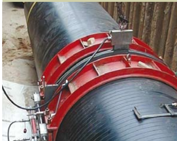
Butt fusion joint - DN/ID 1400mm
