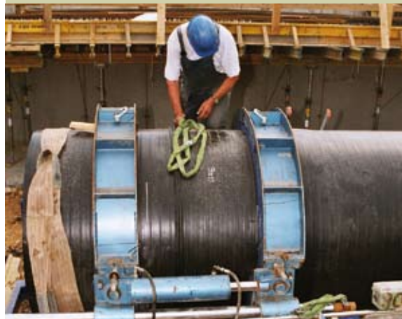
Butt-fusion of a Krah-Pipe DN/OD 1600 mm SDR17
